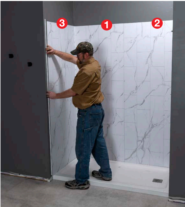
Install the J-trim to cover the outside edge of panel 3.
