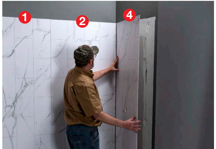
Apply sealant into the other side of the inside corner trim that is already installed. Then apply adhesive to the back of panel 4 and affix to right wall and making sure it is inserted into the inside corner trim.
