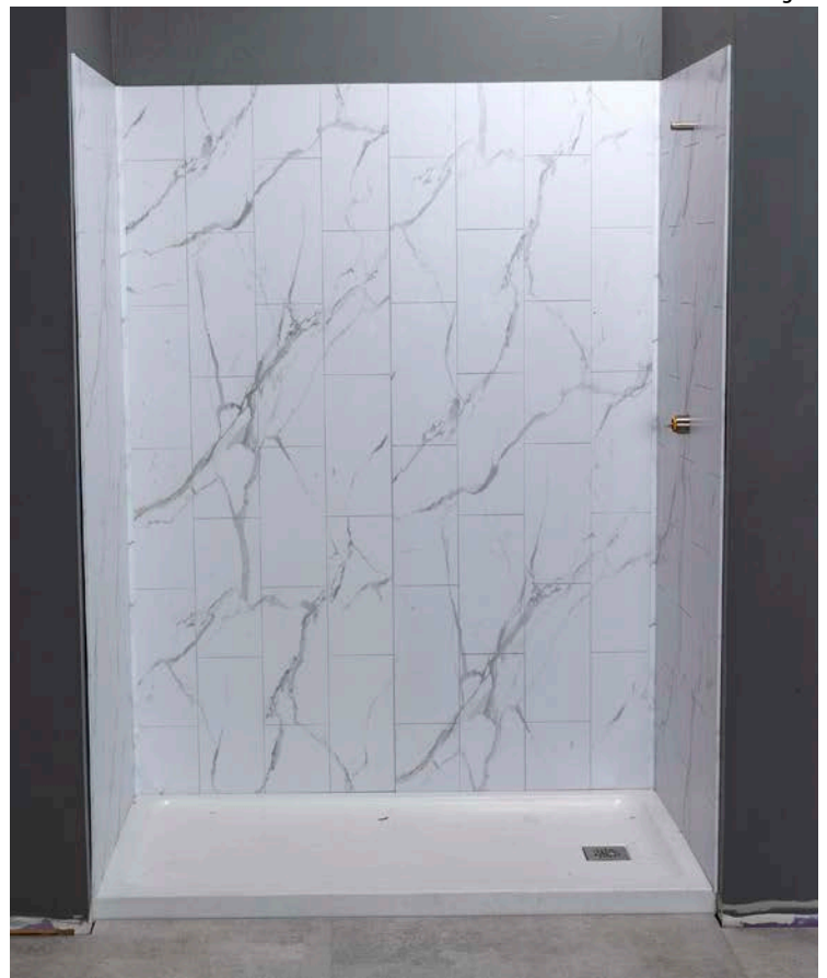
Completed shower wall system install.
