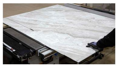
Measure and cut wall panel according to desired size. A table saw is recommended for cutting larger lconic panels. High-grip construction gloves are also recommended, as dust from cutting can make panels harder to handle.
