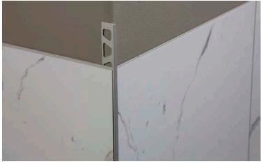
An aluminum tile edge piece, which can be found at most home improvement stores, can be used for a clean connection at outside corners.
