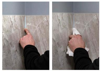
Apply more sealant to front of panel as necessary. Wipe off excess with a soft cloth. Do not use paper or shop towels, as they could scratch the surface of the panel.
