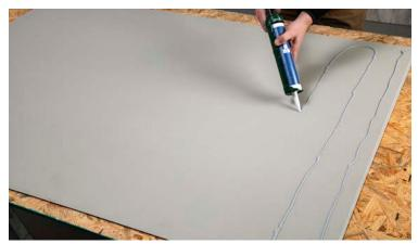
Once tiles are cut, apply adhesive to the back of the panel. Using recommended adhesive, apply a 1/8" bead around the perimeter of the panel, about 1" in from the edge. Then, apply rows of adhesive every 4-6" apart in a typical "M" or "W" pattern.
