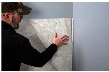
If using lconic panels in a wet environment, apply a 1/8" bead of sealant to the wall about 1/4" in from the corner. Slide the panel into the corner over the sealant.
