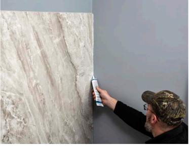
Then, apply a second bead of sealant over the panel at the inside corner of the wall. This second bead ensures a watertight barrier, preventing moisture from getting behind the panel.
