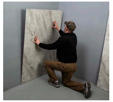
Apply the panel to the substrate by pressing it into place. Apply even pressure with your hands across the entire panel. If necessary, use shims or pins to hold panels in place until the adhesive sets.
