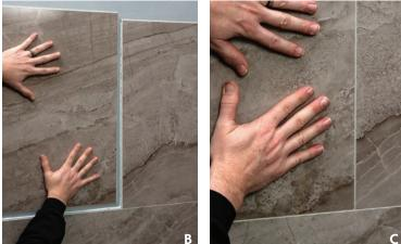
Installation in environments exposed to a direct flow of water (shower, mud room or garage) require a 1/8" bead of sealant to be used in all tongue and groove connections (image A). Add a bead of the sealant along recently cut edges to be placed into the corner. Repeat this process on perpendicular panel also facing corner (image B). Slide into place (image C).
