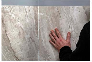
When installing the second and subsequent panels, engage the tongue and groove connection and move panel into place.
